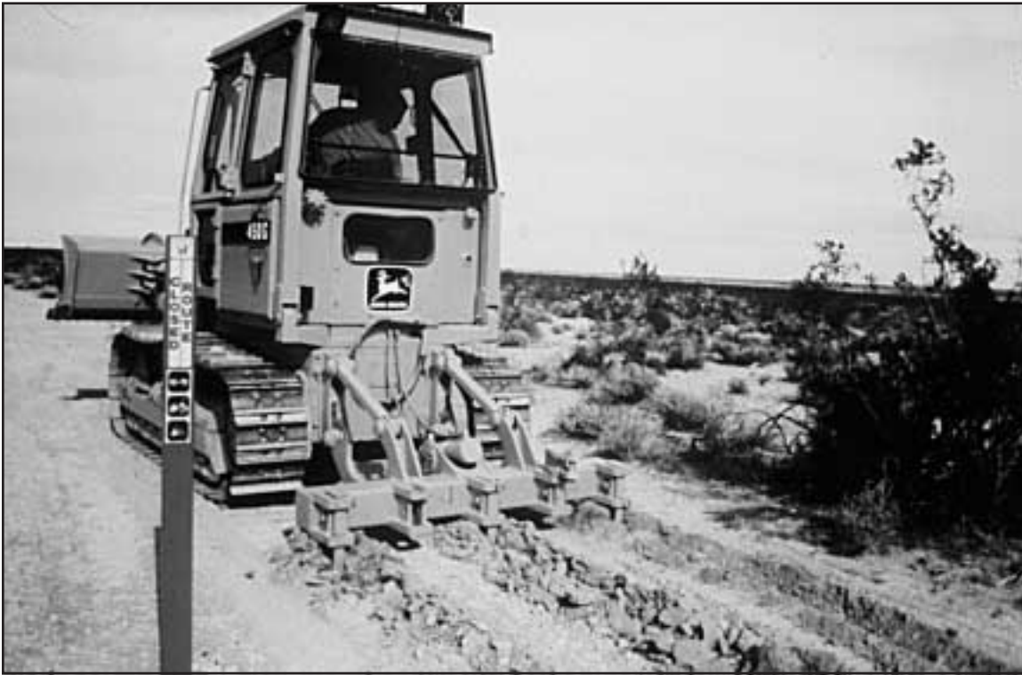
Road-ripping in the Fremont Valley, Mojave desert, California. Photo courtesy of Southwest Center for Biological Diversity.
