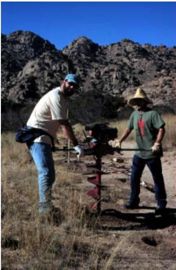
Using an auger to decompact a desert road on the Coronado National Forest.
