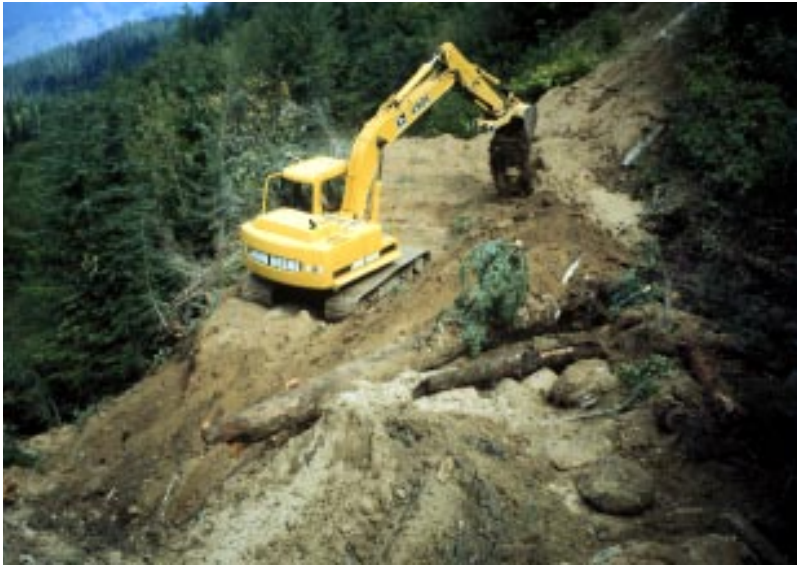
Pulling fill from a road slope.
