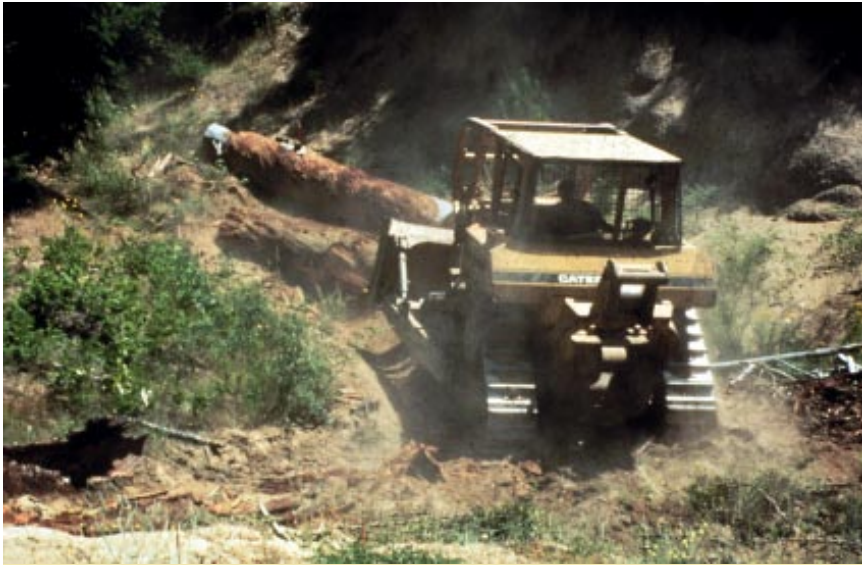
Heavy equipment plays a leading role in road removal.
